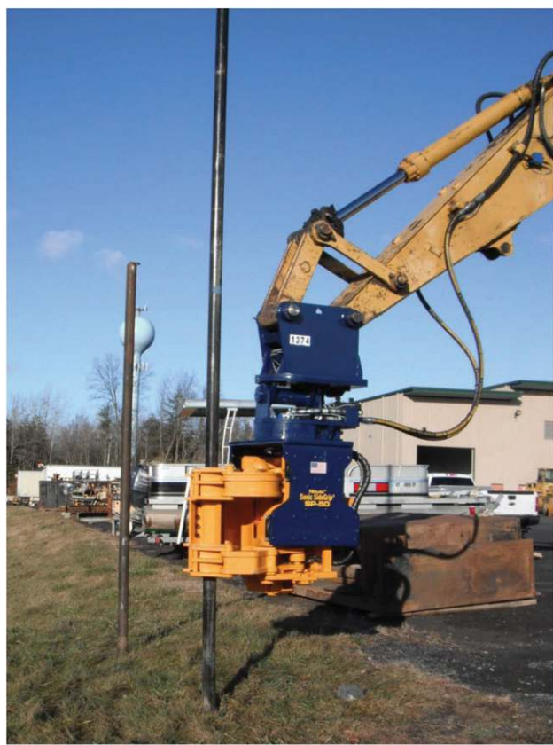
Figure 4. Direct-drive installation of ISTD heater casing.
