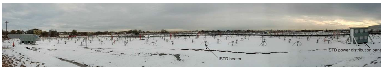
Figure 7. ISTD well-field in operation during New Jersey winter.
