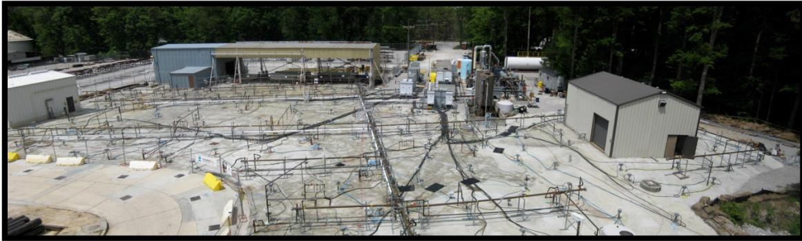
**Project Information:** A combined In Situ Thermal Remediation approach utilizing In Situ Thermal Desorption (ISTD) and Steam Enhanced Extraction (SEE) was implemented at a former vapor degreasing facility and leach pit at Arnold Air Force Base in Tullahoma, TN (Solid Waste Management Unit 10 [SWMU-10]). An estimated 31,000 gallons of chlorinated solvents (primarily PCE) were disposed of at SWMU-10, posing a regional risk to groundwater.
