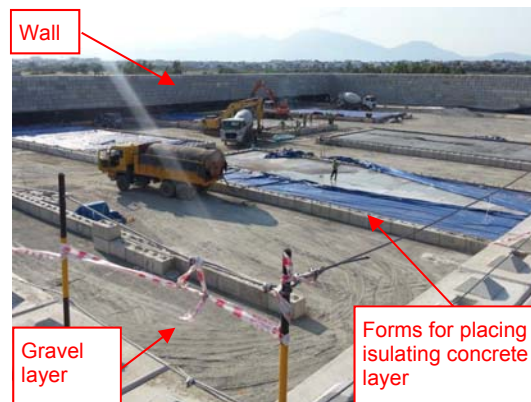
Foundation of the pile containment structure (Photo: CDM Smith)
