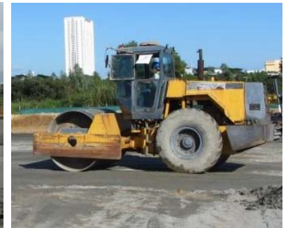
Compacting fill material (Photo: CDM Smith)
