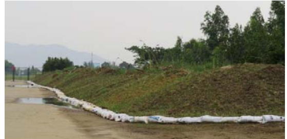
Stockpile of approximately 250 m 3 of clean topsoil material being composted (Photo: CDM Smith)
