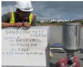
Sand cone testing of compacted fill material (Photo: CDM Smith)
