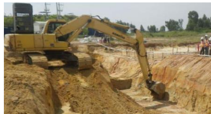
Excavating the former Drainage Ditch (Photo: CDM Smith)
