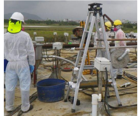
Collecting post-treatment samples from the thermal treatment structure
