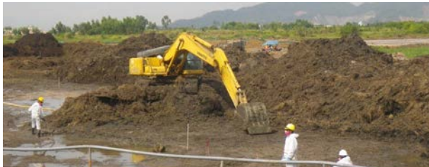
Excavating contaminated sediment in Sen Lake (Photo: CDM Smith)
