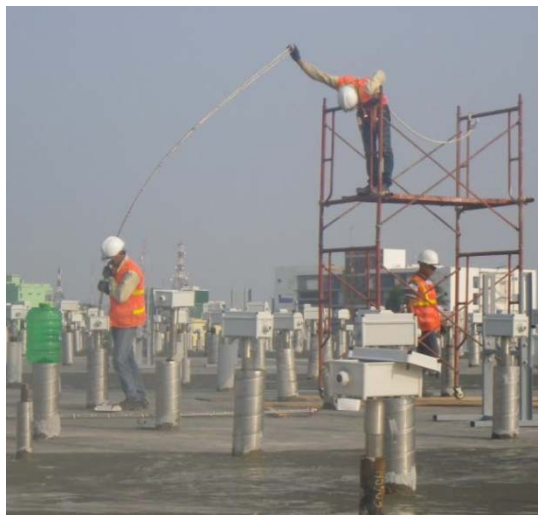
Installing heating elements into heater wells (Photo: CDM Smith)
