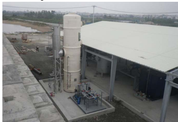
Liquid/vapor treatment plant construction (Photo: CDM Smith)
