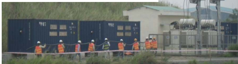
Installing power cables
