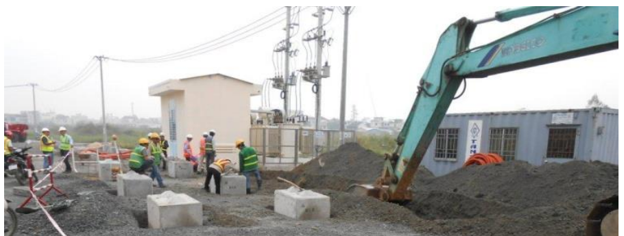
Installing electrical conduit to power the treatment system (Photo: CDM Smith)
