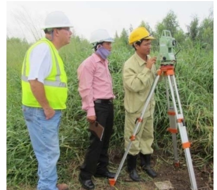
Surveying excavation limits (Photo: CDM Smith)
